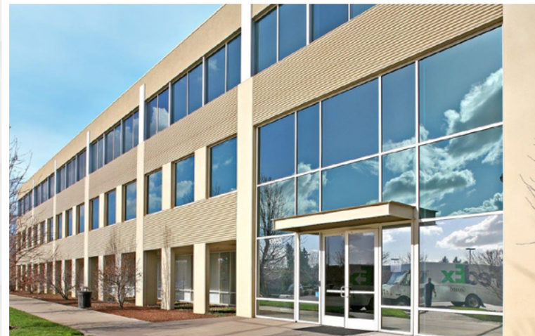
BUILDING E (EXPLORE) 10850 GOLD CENTER DRIVE
