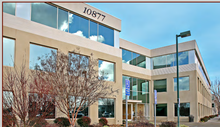
Building D esign 10877 White Rock Road
